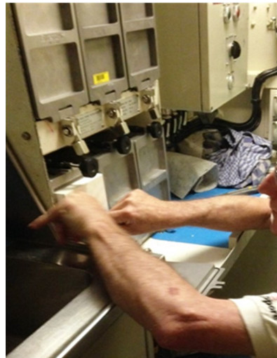
PowerCube ® being installed into canister
