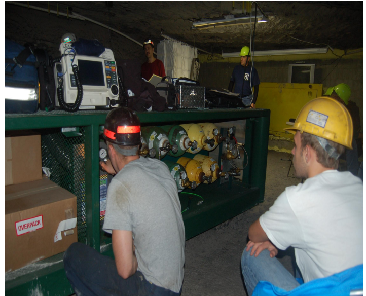
FIGURE 2 MINE LIFELINE BREATHABLE AIR REFUGE
